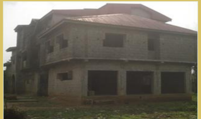
Our maternal and infant hospital under construction needs your help
